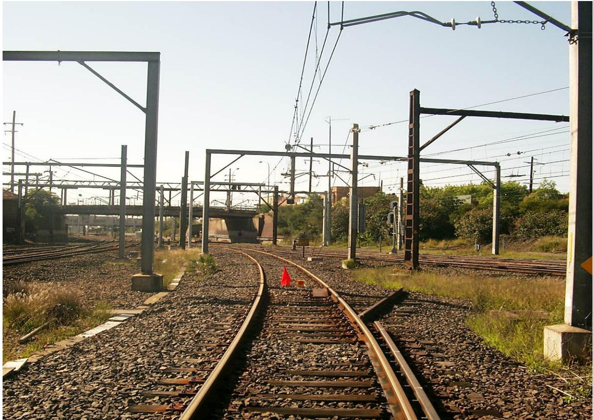
Picture 2: Granville 710 catch points, located on Down West Main showing the proximity of Up South Line and OHWS. Picture taken with back to Country.
