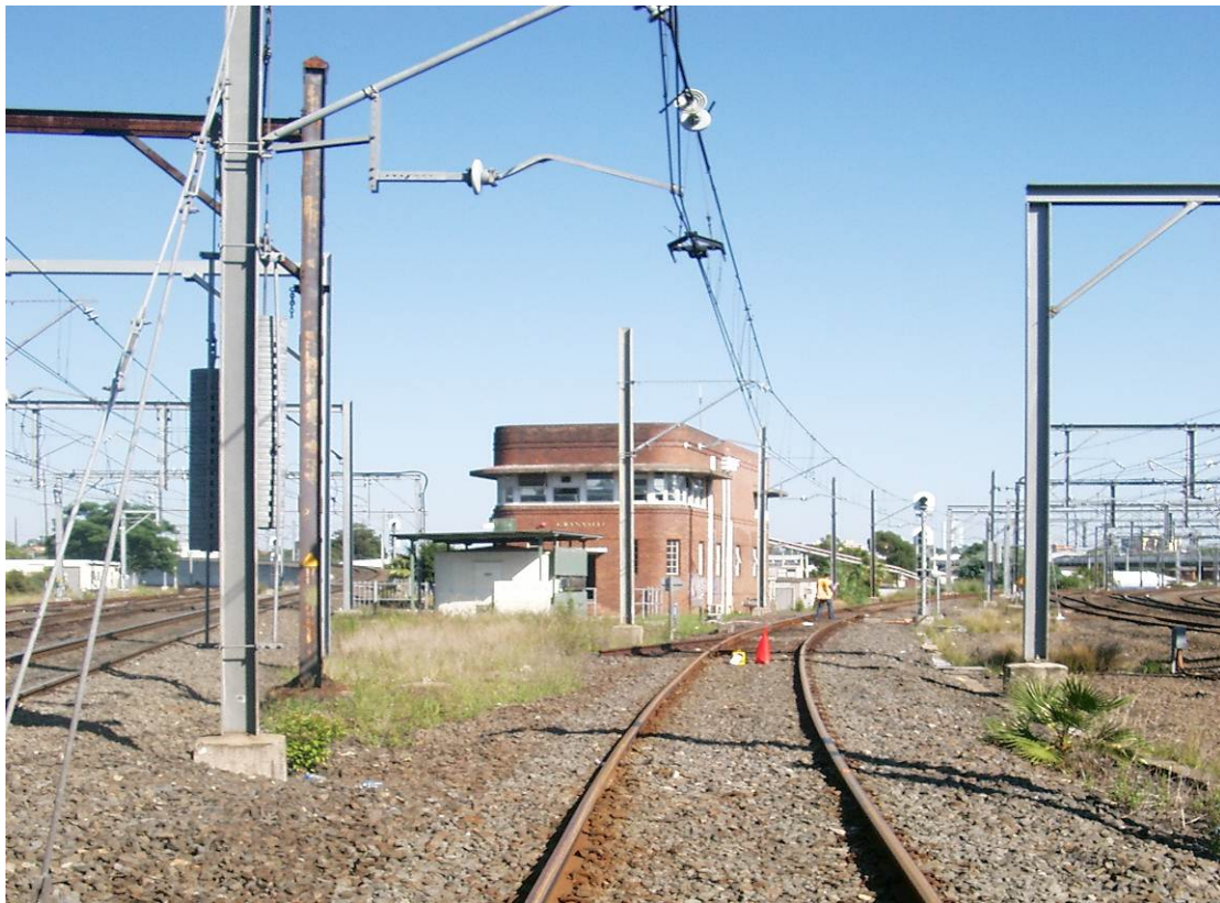
Picture 1: Granville 710 catch points, located on Down West Main showing the proximity of Up South Line, OHWS and Signal Hut/Box. Picture taken with back to Sydney.
