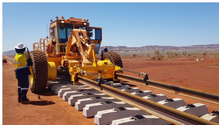
Figure 11 - Pettibone performing rail unloading on Gudai-Darri
