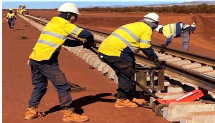
Figure 12 - Trial of Trolley Jacks on Gudai-Darri
