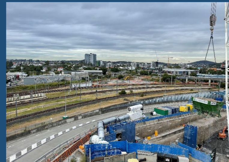
Cross River Rail Brisbane Project Management & Constructability
